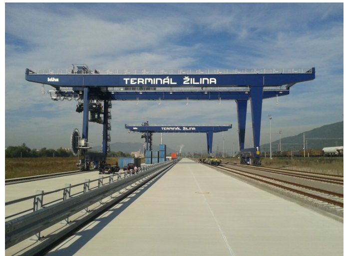
Fig. 1 Rail mounted gantry crane in Zilina ITT, Slovakia. Source: authors
