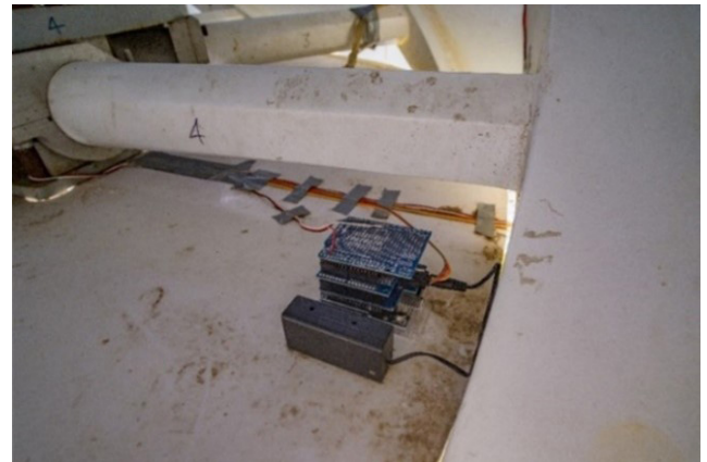
Fig. 10 Arduino microcontroller installation
