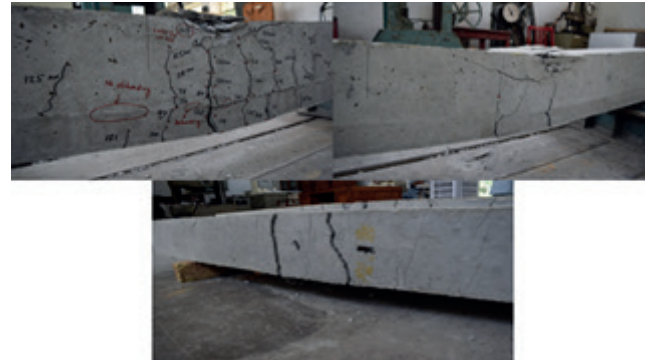
Fig. 15 Cracks formation and their distribution in RECC 75 beam
