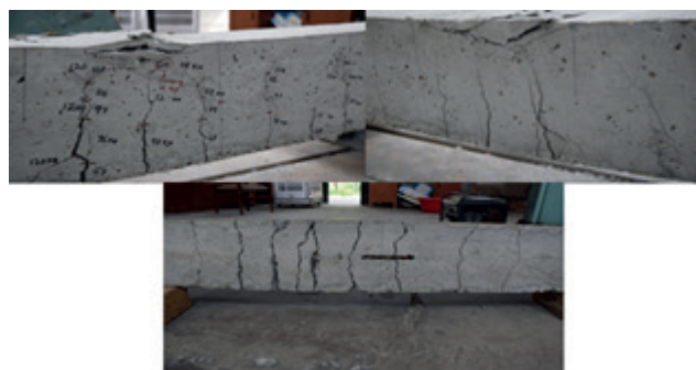
Fig. 13 Cracks formation and their distribution in RC- control beam
