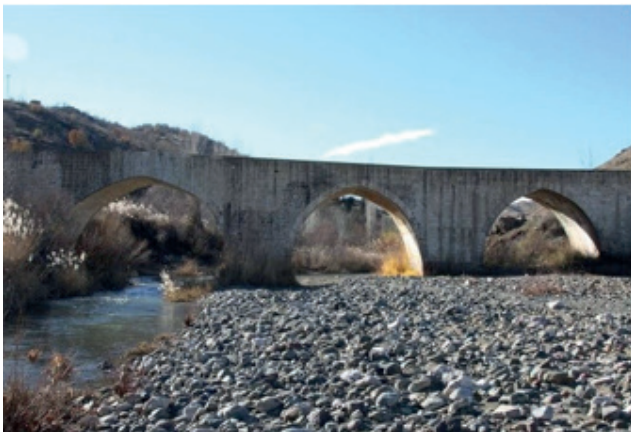
(a) Downstream view
