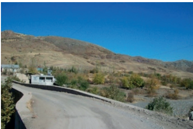
(c) Bridge floor
