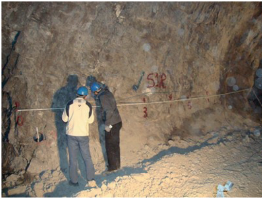
Fig. 3 Mapping of fractures using scanline method in Rudbar Lorestan dam site cavern
