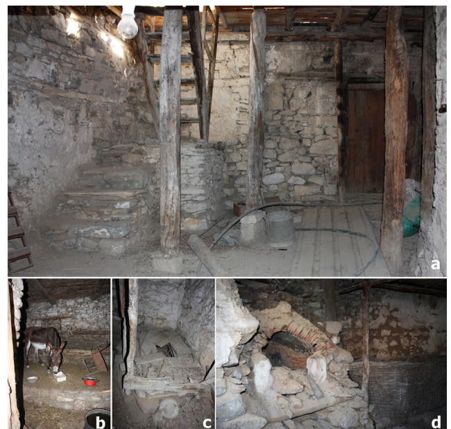
Fig. 17 (a) Spatial organisation of Taşlık space, (b) a Taşlık including barn, (c) toilet, (d) fireplace and basket
