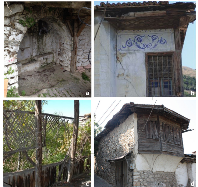
Fig. 15 (a) Fountains carved into the base, (b) Kalem işi below the eaves, (c) lattices, (d) brackets supporting the first floor
