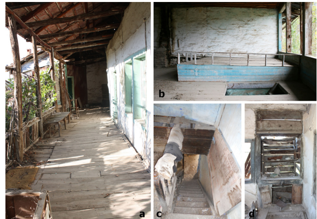
Fig. 18 (a) The view of Hayat ; (b) a Hayat including köşk , (c) staircase and its shutter, (d) abdeslik
