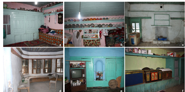
Fig. 19 (a) A room including fireplace, (b) sedir , (c) cupboard, (d) tahtabaşı , (e) gusülhane , sedir and tahtabaşı , (f) counter
