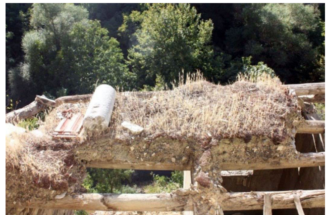
Fig. 8 A terrace roof finished with earth
