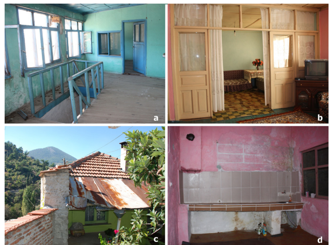
Fig. 24 (a) The conversion Hayat into a room, (b) the conversion semi-open Hayat into closed space with additional timber wall, (c) mass addition for service necessities, (d) the conversion room into a kitchen
