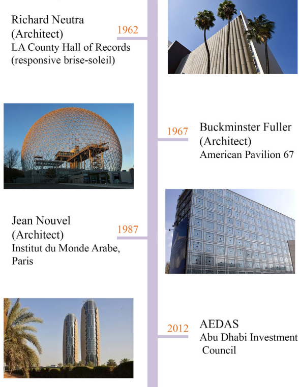
Fig. 5 Examples of kinetic façades, responsive to the surrounding environment (prepared by the author)
