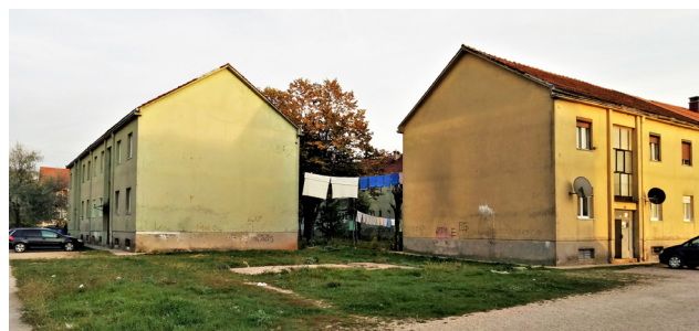
Fig. 10 A view on typical One-storey buildings (Bojković, 2020)
