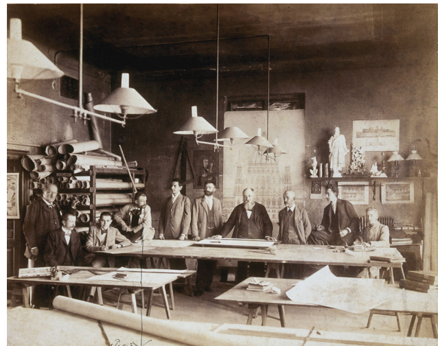
Fig. 6 Imre Steindl among the employed architects in the on-site office, photo of Károly Divald, Jr., 1896 (Source: MÉM-MDK, without inv. no.)
